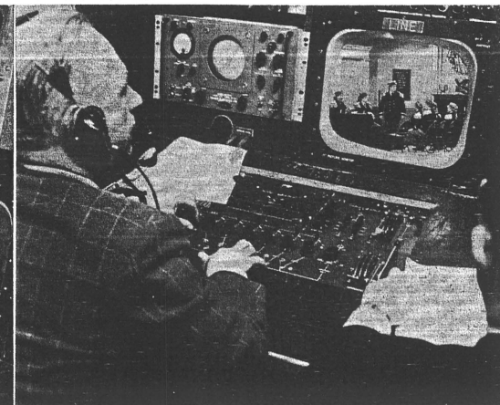
PICTURE on "line" monitor is the take selected for kinescoping, will be included in finally edited version of the show. Effects are added to kinescope electronically, duplicated in edited film.
